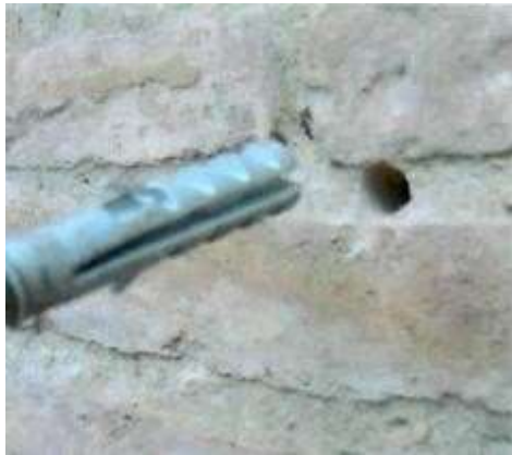
Figure 10 - cleaning the hole and inserting expansion plug
