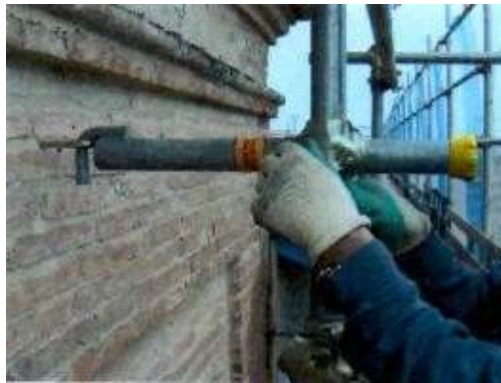
Figure 12 - mounting anchor with tube and clouper
