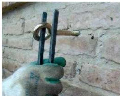
Figure 11 - screwing the eyebolt
