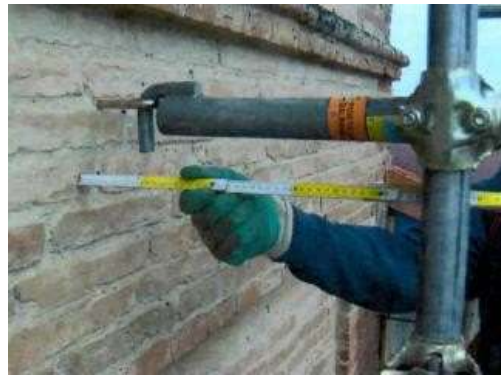
Figure 13 - control of the exact distance from the wall
