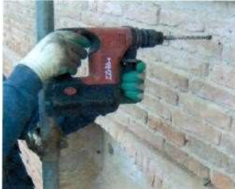
Figure 9 - drilling of the wall support with electric drill
